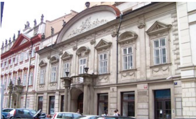
Historical building, offices Prague CZ, 2015 - CoolGRID
