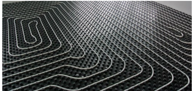
Figure 9 Underfloor heating pipes layout
